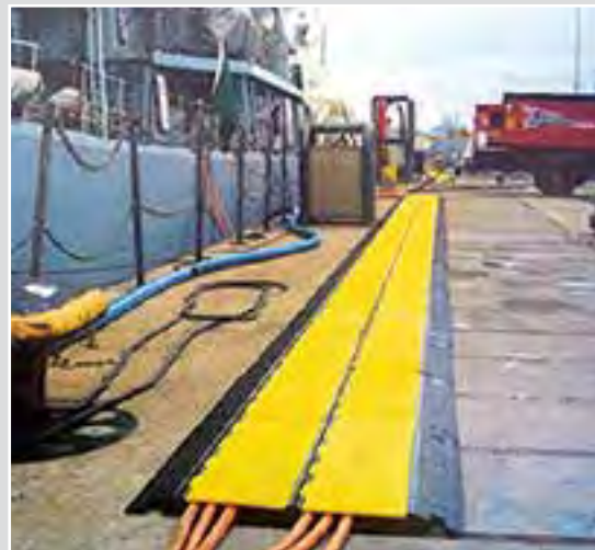
AMS in use at Naval dock yard
